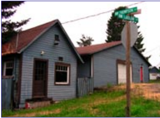
Former Bonny Slope barbershop and store at Laidlaw & Thompson
