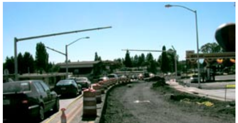
Westbound Cornell - preparing the grade with curbs and sidewalks in place
