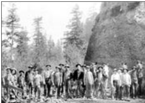
Work crew repairing Cornell Road, circa 1915
