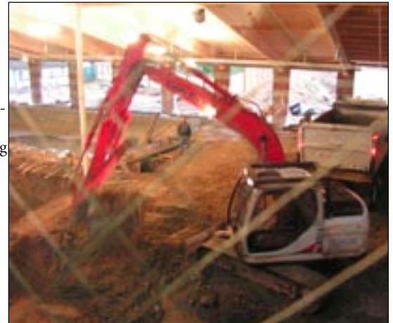
Excavation for the new aquatic center lap pool
