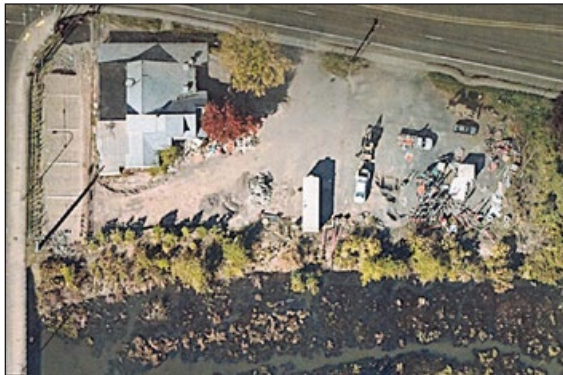
The aerial photo of the lot before demolition shows how close it is to the stream.
