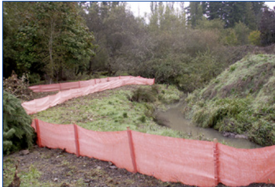
Cedar Mill Creek flows out of what used to be the millpond and runs through a culvert beneath Cornell before it cascades over the falls.
