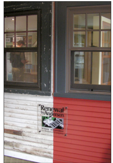
Before-and-after displays in the showroom, provided by RbA, help customers envision how their finished projects will look.
