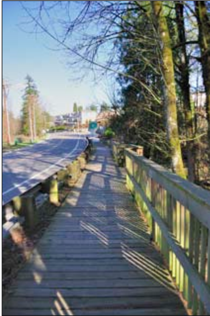
The Larry Vincent Memorial Bridge was rebuilt in 2002 after problems with the 24-year-old wooden bridge were discovered. The new bridge was made with pressure-treated wood and heavy beams salvaged from another bridge on Germantown Road. Photo by Neil Hefty
