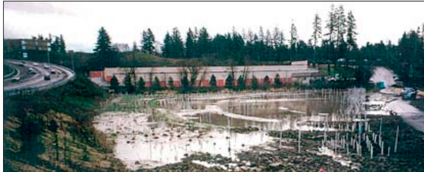
The Center Wetland in February 1997, during initial restoration work
