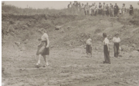
Groundbreaking at the original site in 1953
