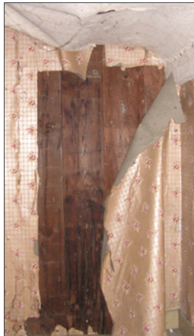
The house is built of vertical 2" x 12" planks of cedar, most likely milled on site. Interior surfaces were applied directly to the planks.
