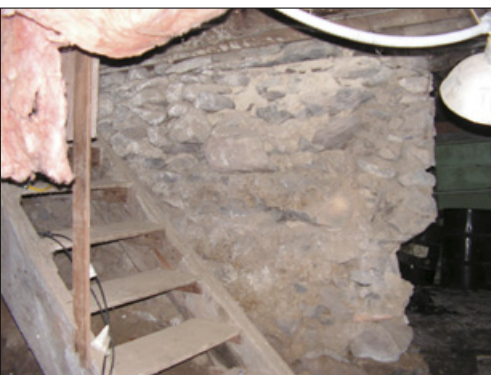
The foundation of the house is a jumble of local stones, bricks and beams, and has to be rebuilt before the house is safe to occupy.
