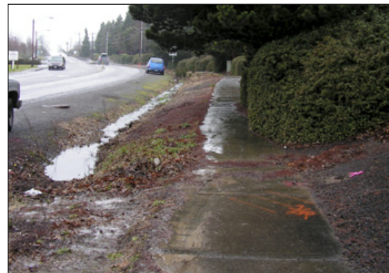
Portions of the existing sidewalk on the north side of Cornell are overgrown with shrubbery.
