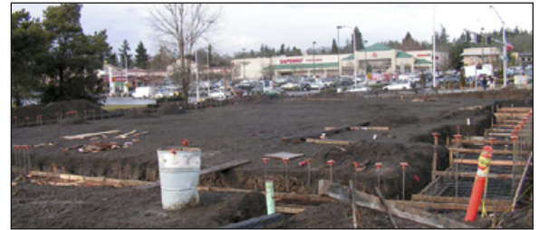
Auto Zone wasted no time in getting underway with the construction of their store. They'll be pouring the concrete foundation soon.
