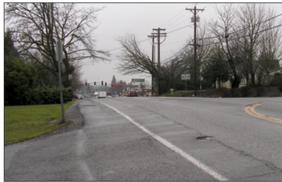
The county believes it has sufficient right-of-way to construct an asphalt path on the south side of Cornell this summer. The Minor Betterments program currently does not include ROW acquisition because it's usually too expensive to meet the $150,000-per-project limit.
