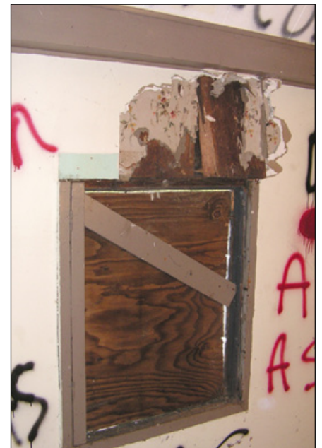
Some of the planks have warped, as around this window in the second floor bedroom. Graffiti adorns the walls from the time before the district obtained the property, when squatters were breaking in regularly.
