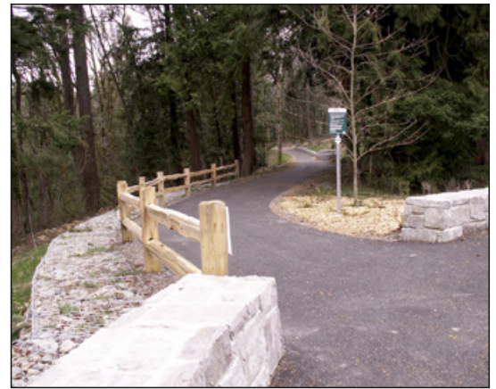
The Husen Park entrance is accessible and provides a wide path that leads to an overlook area.
