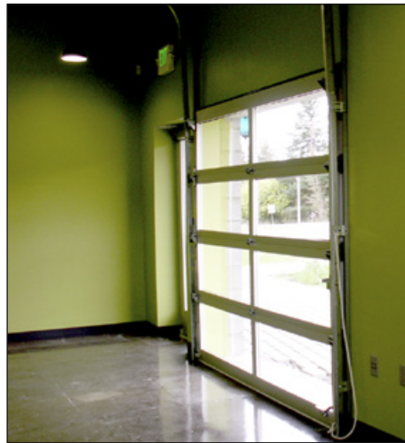
Behind a roll-up door at the front of the building is a space reserved for a future retail business, probably something like a small café or ice-cream shop.
