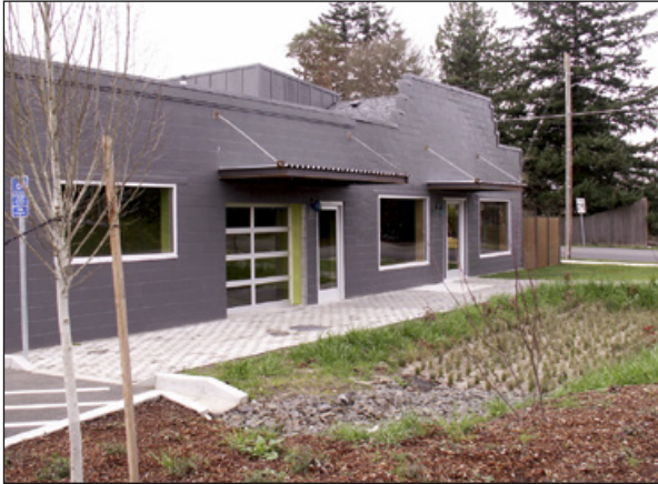
There were many conditions attached to the permits for remodeling the building, including "half-street improvements" to the intersection, sidewalks, and a water-treatment swale to catch runoff from the parking lot. But the new owners felt the requests were appropriate and added to the property's value.
