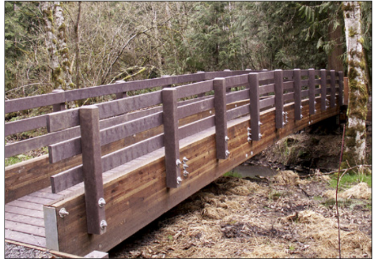
A wood and composite bridge spans Cedar Mill Creek.
