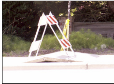
The buckled sidewalk on Saltzman may lead to a change in Oregon law.
