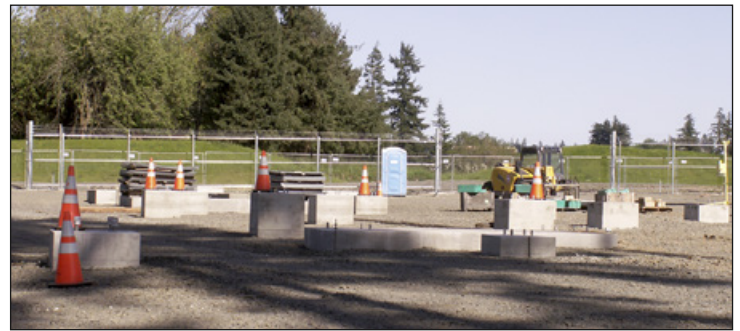
A new PGE substation is being constructed between Highway 26 and the Commons at Cedar Creek apartment complex. No word yet from PGE about a completion date or the area it will serve.
