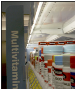
LED lighting is featured throughout. Bands of tiny LEDs shine from the shelves directly onto the products, so light isn't wasted, and items are easy to spot in the clear, energy-saving, natural-color light.
