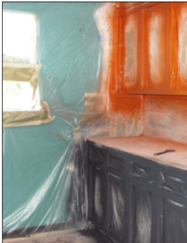
After masking all non-treated surfaces, cleaning and sanding the boxes, several coats of paint were sprayed onto the cabinets. Doors and drawer fronts are being refinished at the workshop.
