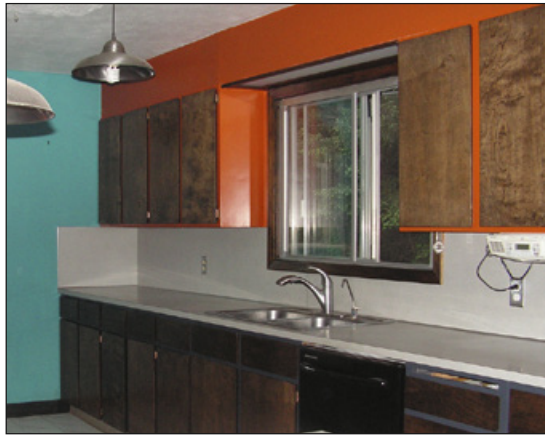
Doors and drawer-fronts refinished, cabinets painted, Mid-Century style!
