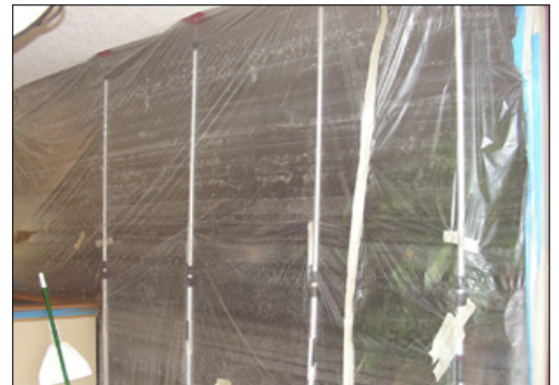
Plastic sheeting protects the rest of the house
