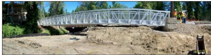
The aluminum bridge for the Laidlaw project was built offsite
