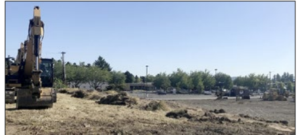
Grading is finally underway. This upper section will include parking for the Sunset Athletic expansion and the shops and offices on the second floor of the east building.
