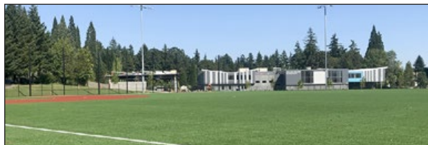
Looking across the artificial turf multi-sport field toward the new William Walker Elementary School
