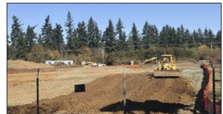
The parking lot adjacent to the Sunset Transit Center is under construction. Peterkort Company said they don't know when it will be open.
