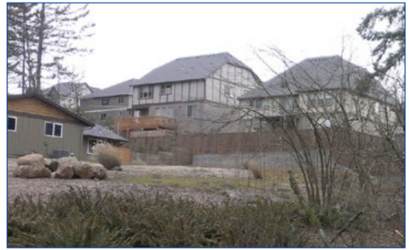
The existing house, left, has lost its privacy when larger homes were built on graded land above it.
