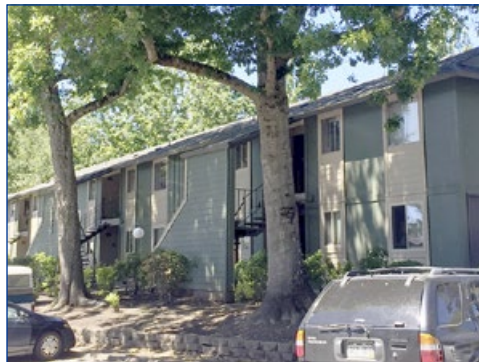
One of several buildings that were renovated under a previous board. Consultants said the repairs were inadequate.
