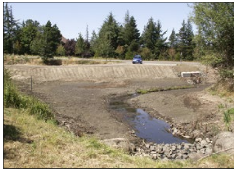
Replanting began as soon as excavation was complete. The green sprayed material now visible is the "hydro-seed."
