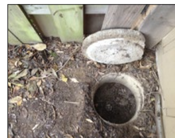
A water shutoff valve in a clay pipe
