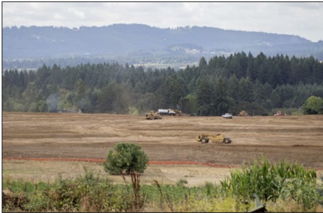
The district's new high school is being built at the southwest edge of the district in an area that is mostly rural now.
