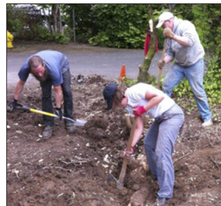
Church members began by removing trees and grading the area
