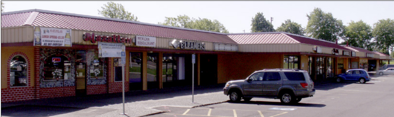
The east end of the Cedar Mill Place Mall is where the new Walgreen's store will go. Tenants will move to the west end as soon as the remodeling has been completed by Tandem.
