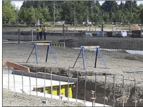
Excavation for infrastructure is underway now
