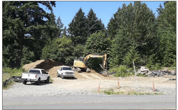
People were speculating that a road was being pushed through here but it's just preparation for utility work for the Life Time project.
